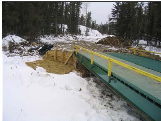
Commercially available steel two piece portable bridge installed on Papineau Road.
