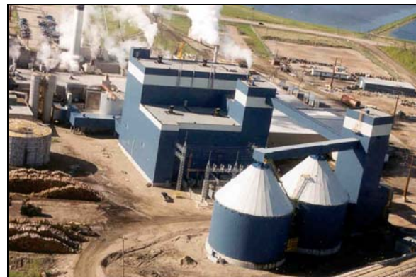
Newsprint Mill Thermo-mechanical pulping (TMP) facility constructed in 2001.
