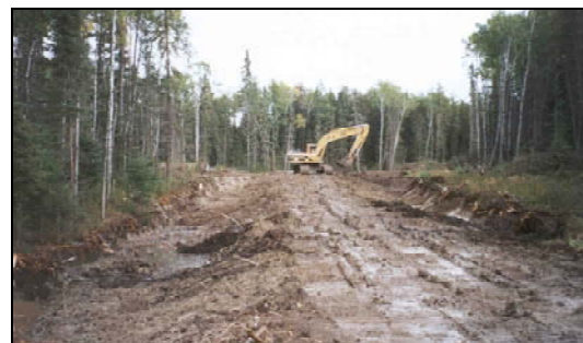
Hollow Water First Nation road construction operation.
